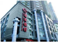
Construction Outer Wall
